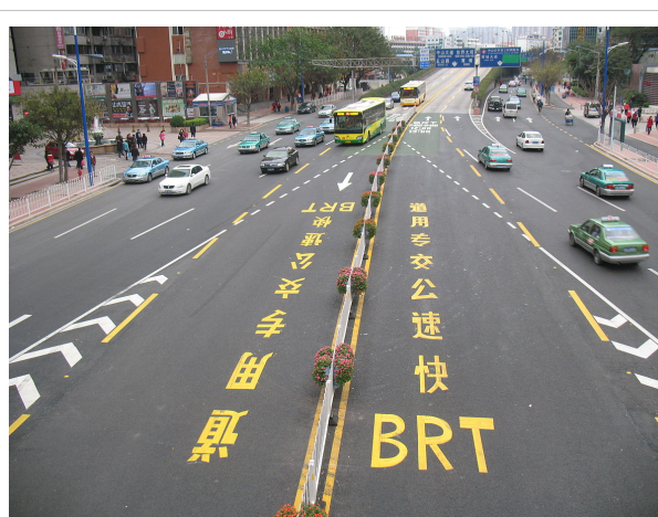
GBRT dedicated corridor
