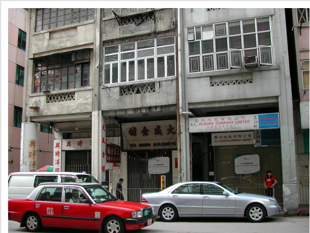
Old-fashioned shops ( tong-lau ) in Wan Chai are typical examples of Lingnan architecture, comparable to those found in Guangzhou and Taipei. Attached to the second storey from the pavement, numerous pillars were built in front of the closed stores.
